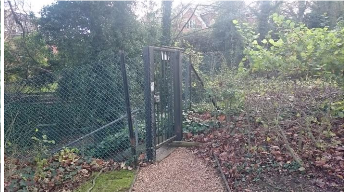
Gate leading to steps
