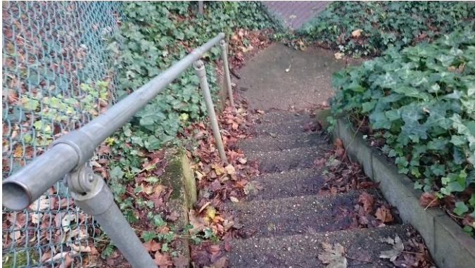
External steps to Chesham Road
