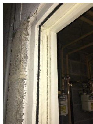
Intumescent strips and cold smoke seals missing
