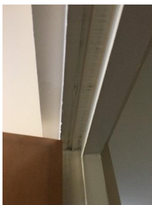
Intumescent strips and cold smoke seals missing
