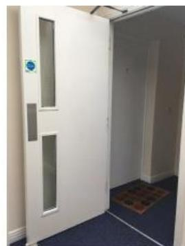
The common parts of Admiral, Charlton & Neville Court have been designed to prevent the spread of fire by ensuring they are clear of combustible materials, and through compartmentalisation, via fire doors. The signage on the fire doors clearly state that they should be kept shut and residents should adhere to this instruction at all times.
